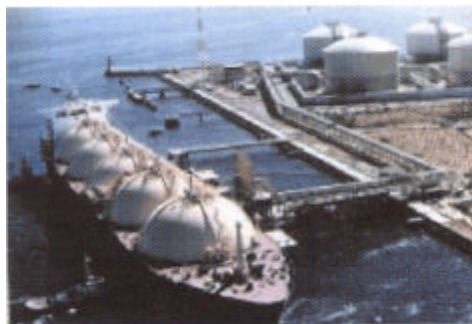
Figura 1. Recepción de gas natural licuado (GNL)
